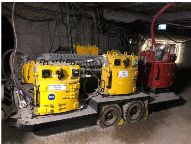
Figure 61 - Station mobile en souterrain
