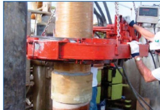
Picture 11 Application of power tong
