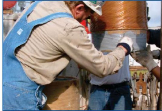
Picture 9: Application of thread sealant
