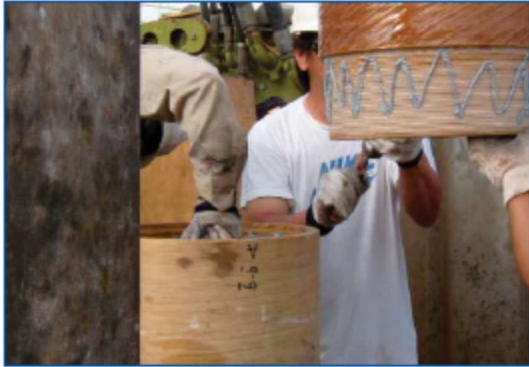
Picture 8: Application of thread sealant
