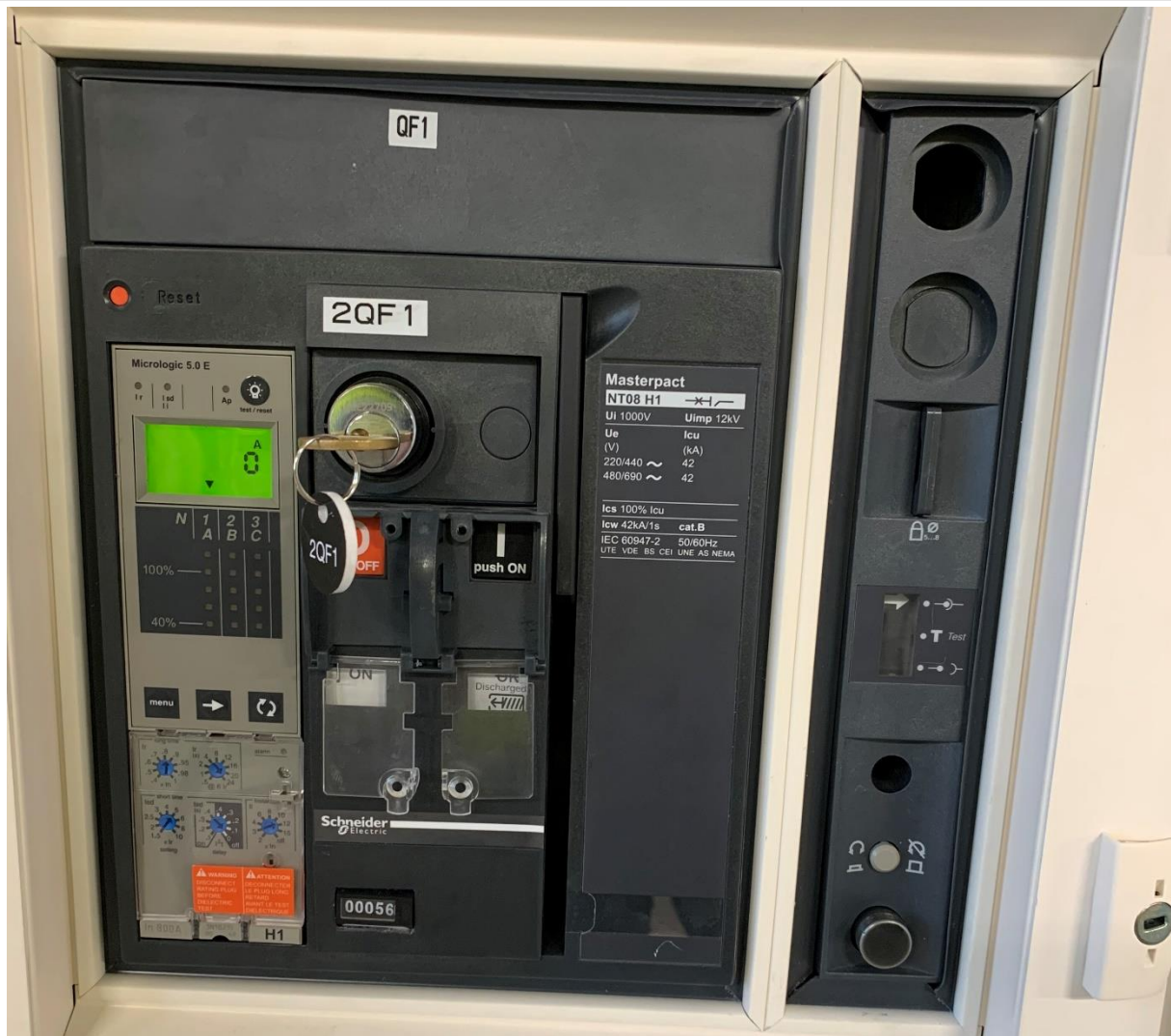
Figure 43 : TGBT 2 – MASTERPACT
