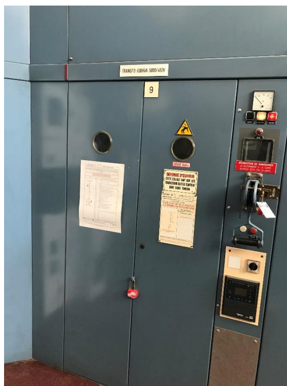
Figure 6 : HTA - Cellule 5kv-460V IT n°9 - Machine JOSEPH
