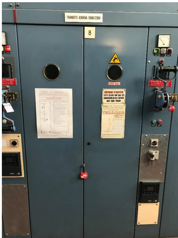
Figure 5 : HTA - Cellule 5kv-220V IT n°8 - Machine JOSEPH
