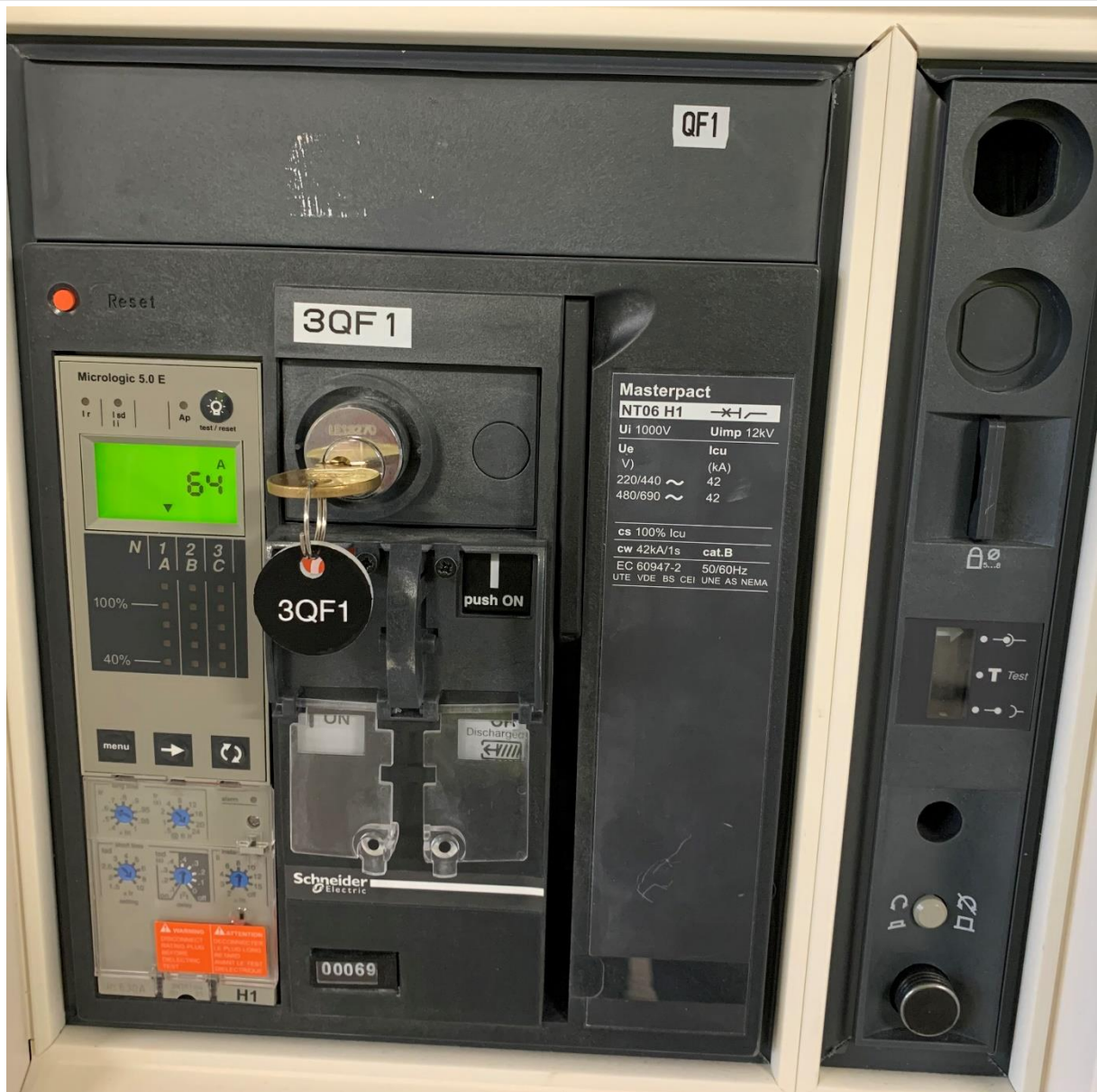
Figure 45 : TGBT 3 - MASTERPACT
