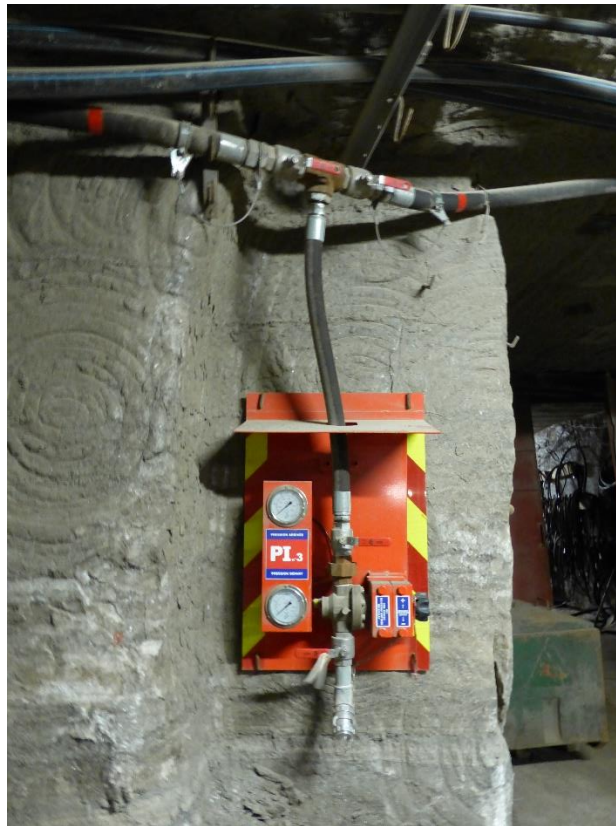
Figure 17 : Platine incendie
